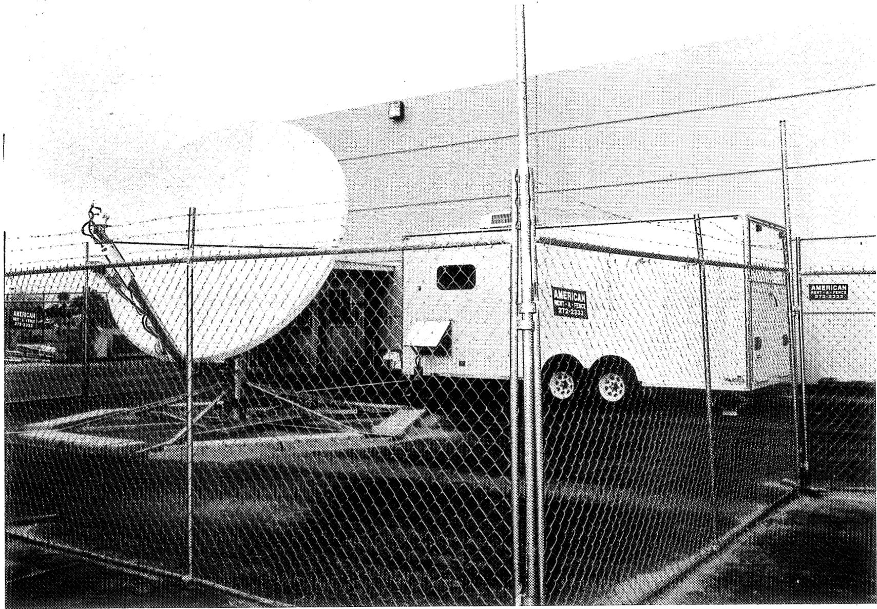
HDR Station at Motorola GSTG, Chandler, AZ 3.4 m, 622 Mbps
