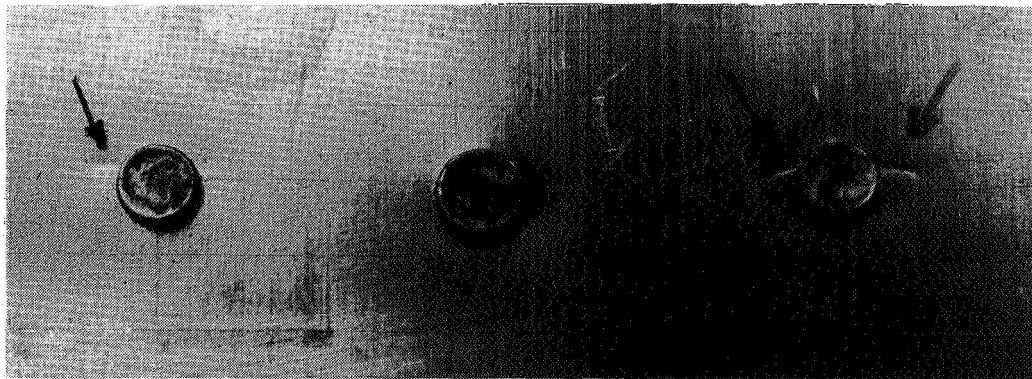
Fig.7 Small cracks at non-countersunk rivet row. These cracks were present after failure occurred at the other critical row with countersunk rivets. (2024-T3 Alclad, t = 1 mm, 3 rows of 7 rivets, d = 3.2 mm, S_{max} = 106 MPa, R = 0 , N = 182000 cycles).
