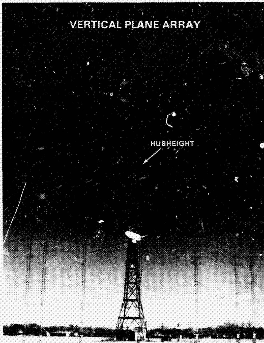
Figure 5--Photograph of PNL seven-tower vertical plane array near the 200 kW MOD-0A at Clayton, New Mexico
