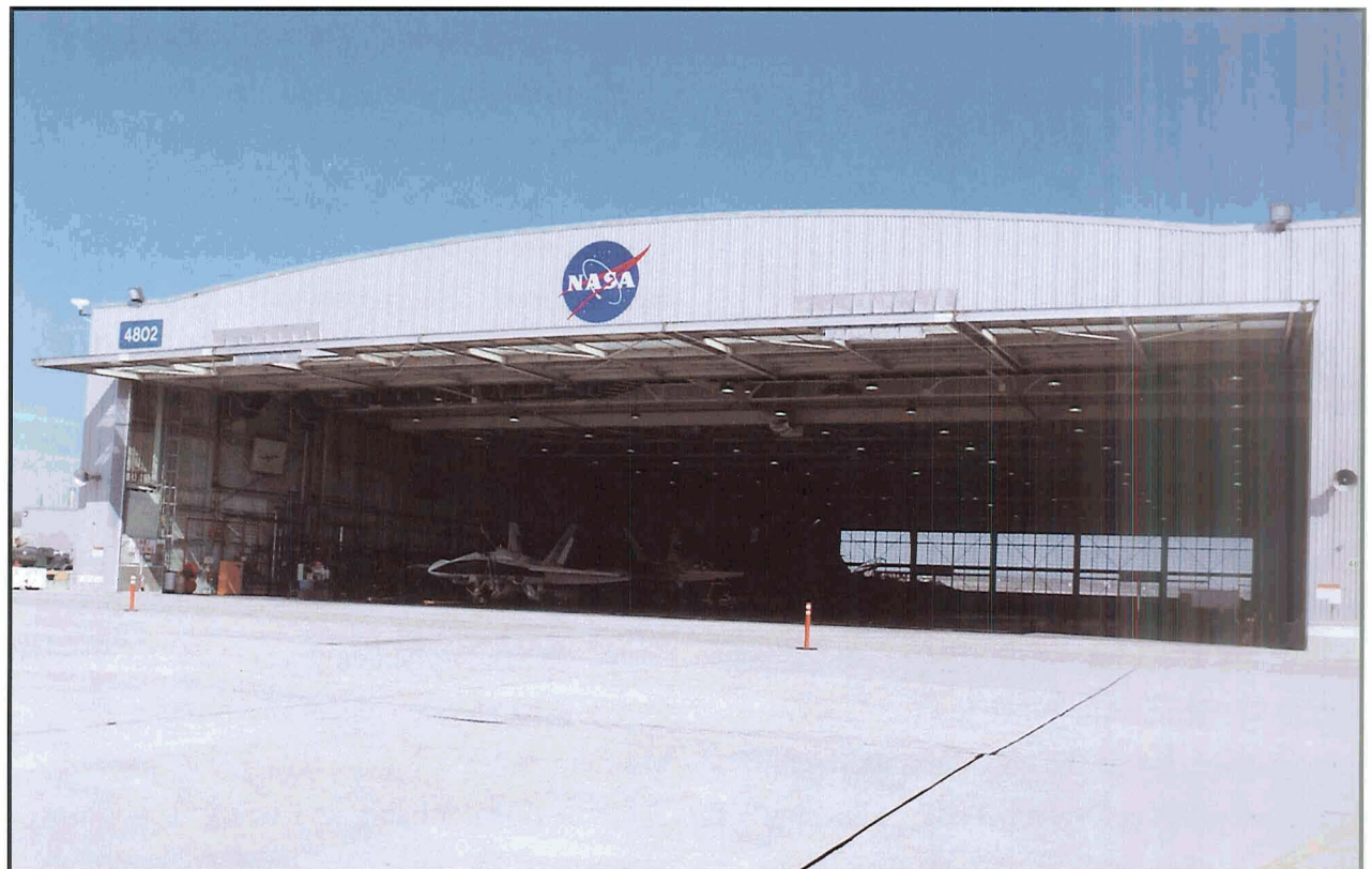
Main hangar at the Dryden Flight Research Center showing a pair of F/A-18s inside (NASA Photo EC95 43079-6)
