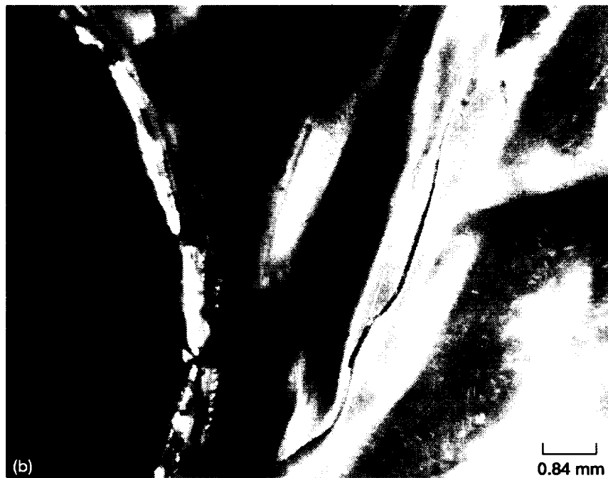
Figure 4. HST MSS MLI near cable holes (16,670 ESH). (a) Extensive cracking of FEP and delamination of FEP from Al (circular area on left). (b) Through thickness crack in 5 mil FEP.
