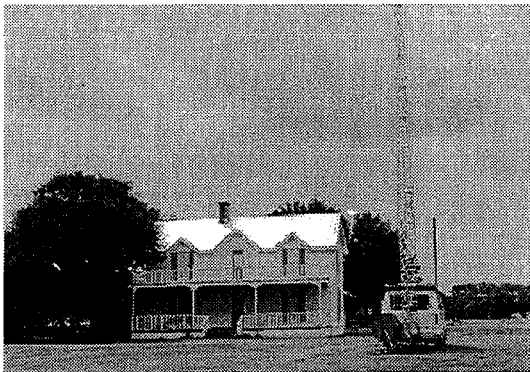
Fig. 1a: The Farmhouse, now with a sheet-metal roof.
