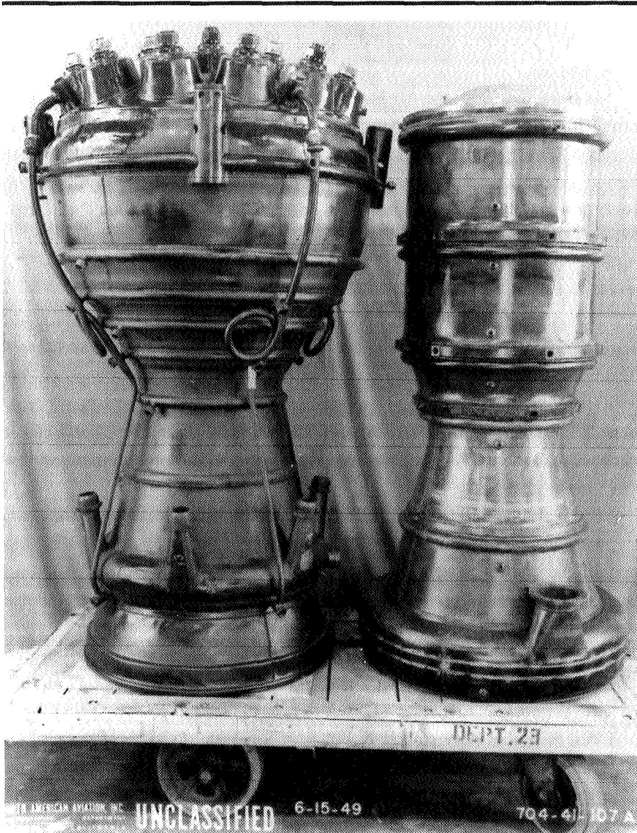
V-2 engine, left, and its successor developed for Navaho. (Rocketdyne)
