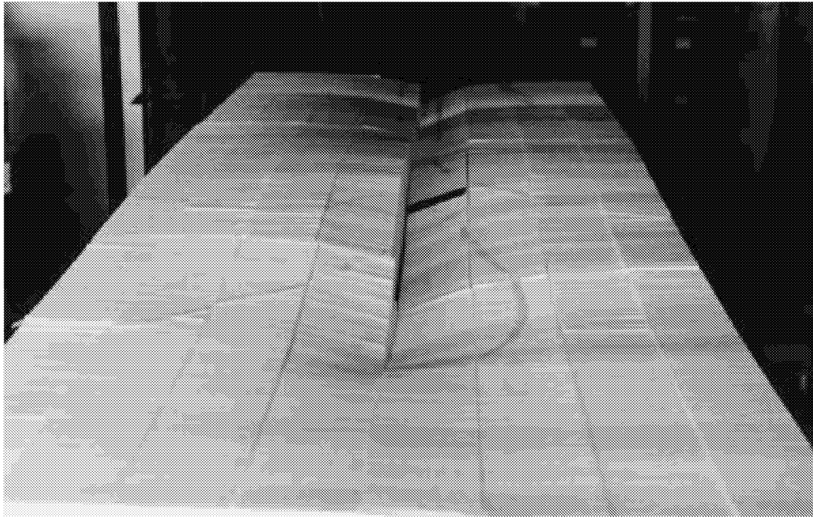
Figure 4. New UWT test section with liner under construction.
