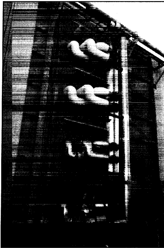
Figure 16. View of the HX coolant supply (smaller diameter) and return (larger diameter) pipes on the West wall of the new C-D leg. Separate pairs of pipes are connected to each of the three streamwise zones in each of the four HX modules that are stacked vertically to form the West HX unit. (C-99-2655)
