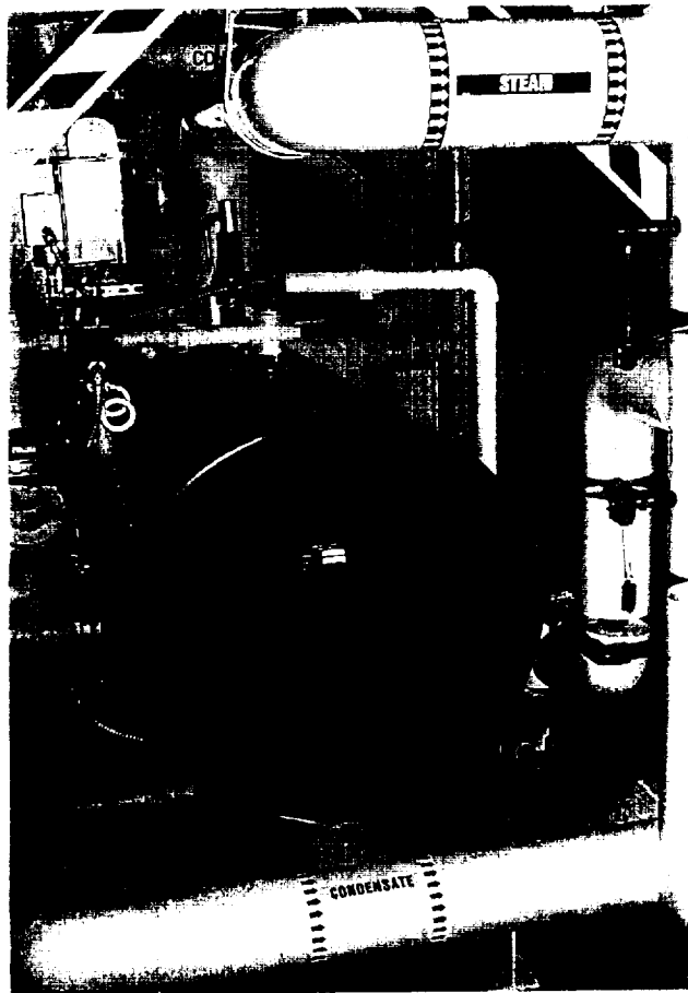
Boiler Assembly at Pad 39-B
