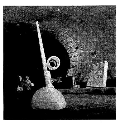
Figure 33: Airframe and Engine Source Noise Testing
