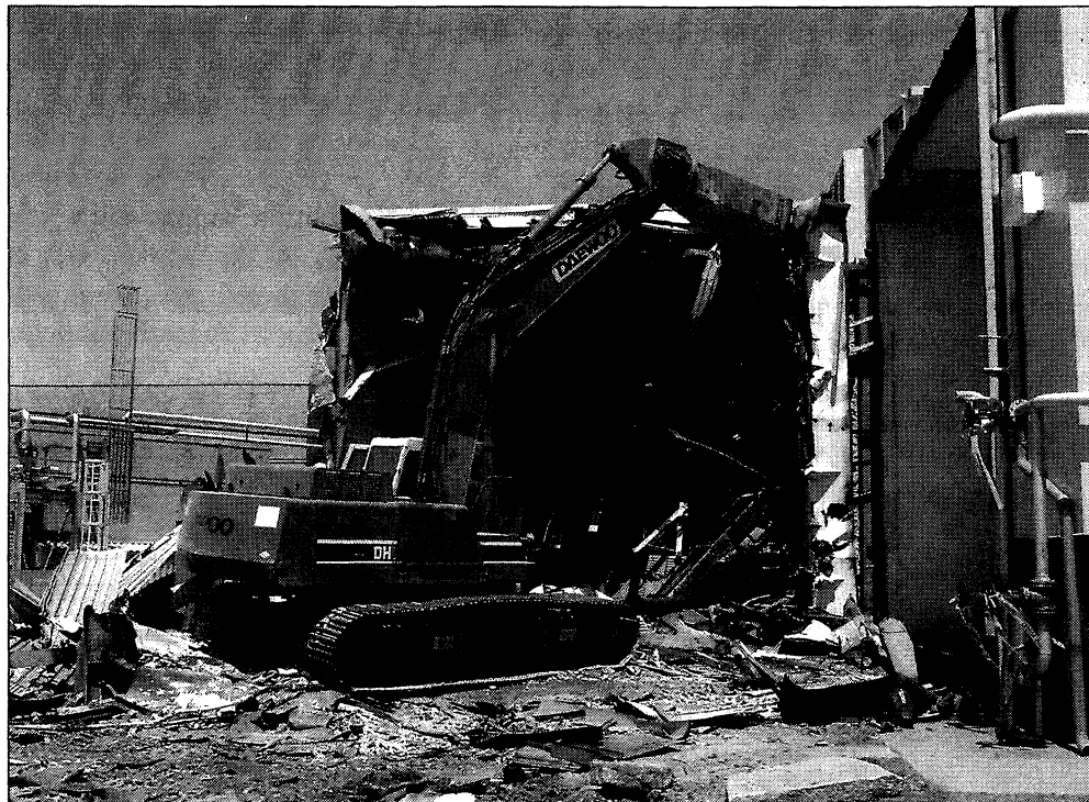
Figure 8-15. Demolition of Corner D and original Carrier heat exchanger, 1999. (NASA C-99-1452)
