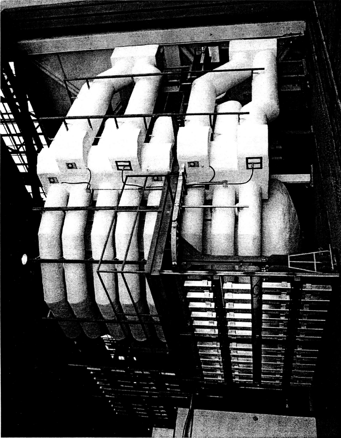
Figure 3. BPC located at Hangar L at KSC, FL (rear view, 1986). (Banks of ballasts for the 96 400-W HPS lamps are visible at the left. Construction began on the chamber in 1985, with operational capabilities completed for most subsystems by 1988.)
