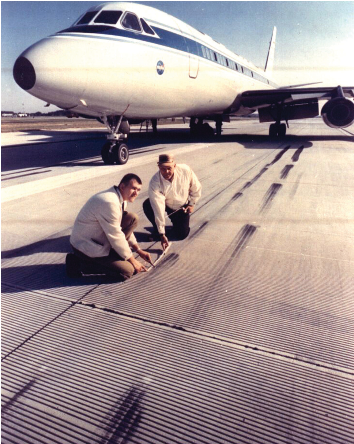
Thomas Yager (left) and Walter Horne inspect grooved concrete surface at NASA Wallops Flight Facility in front of Convair 990 test aircraft. In 1968, these experiments evaluated effectiveness of grooved runway surfaces for safer wet pavement landings.
