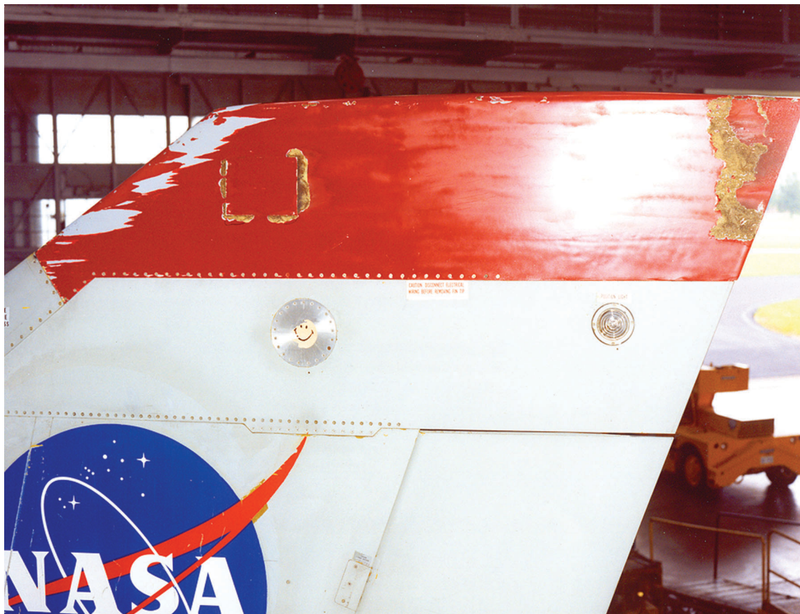
Damage to composite fin cap on F-106B. Note burn areas around inspection panel and near trailing edge of cap.
