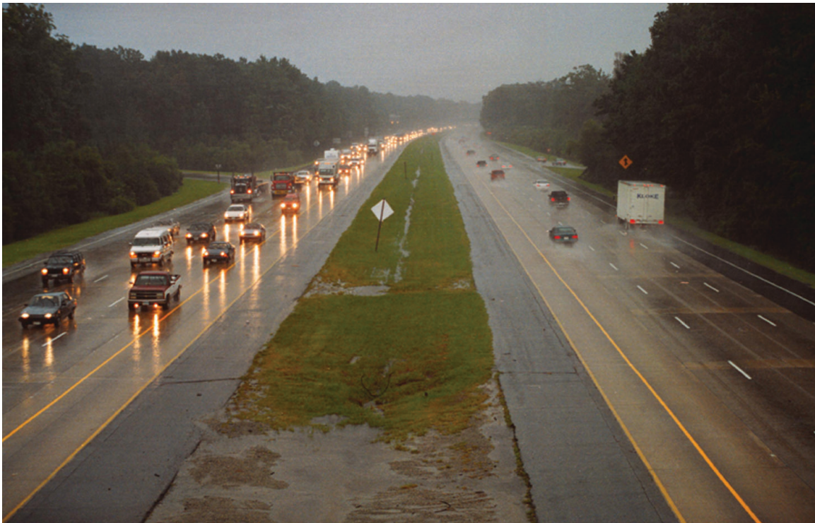
Langley's pioneering efforts on runway grooving have been extended to national highways for enhanced safety in inclement weather.
