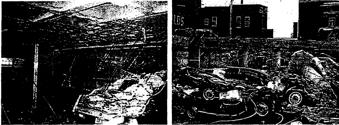
Figures 7a and 7b: Structural damage resulting from corrosion of reinforced concrete buildings [4-5]
