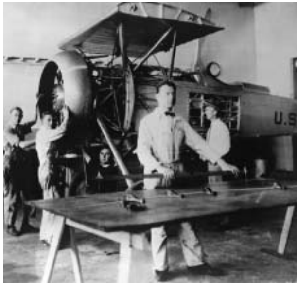
Langley metal workers fabricated NACA cowlings for early test installations.
