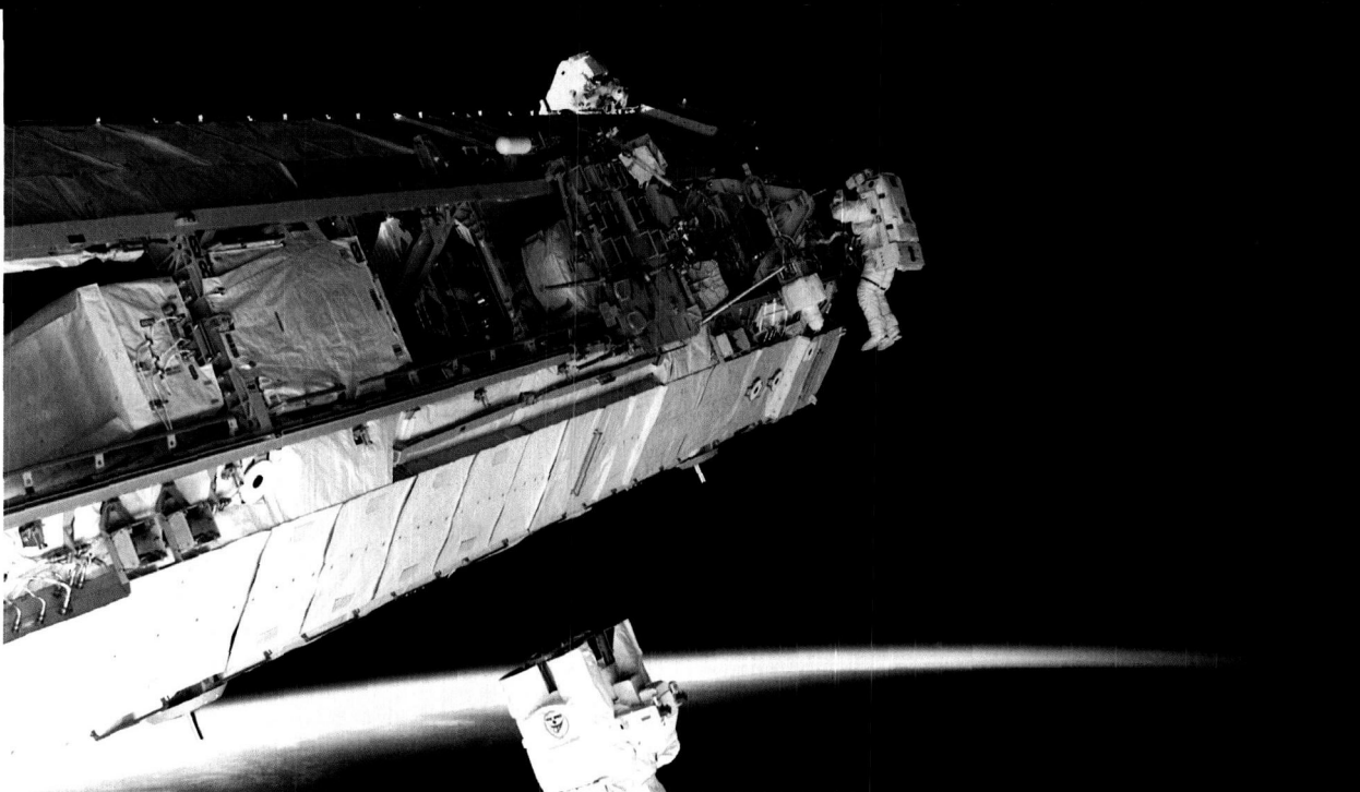
Astronauts Michael Lopez-Alegria and John Herrington install the Port One (P1) truss on the International Space Station (ISS) in November 2002.
