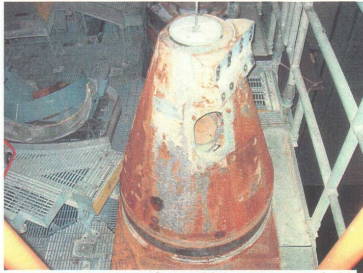
Figure 7. Support post four, which connects to hold-down post four on the SRB.
