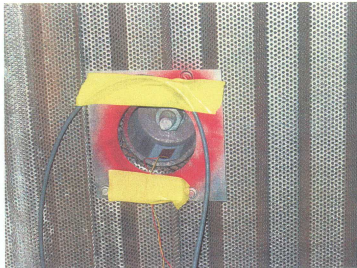
Figure 10. Bolted connection of heat shield pin with MFC sensor installed.
