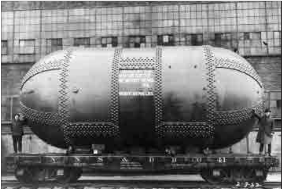
The young NACA first built its reputation as an outstanding aeronautical research institution on the strength of its Variable Density Tunnel (VDT). The tank for the VDT arrived at Langley by rail from its manufacturer, the Newport News (Va.) Shipbuilding & Dry Dock Company in February 1922. It was an eighty-five-ton pressure shell with walls made from steel plate lapped and riveted according to a practice standard in steam-boiler construction. NASA Image #L-1990-04352 (LaRC)
