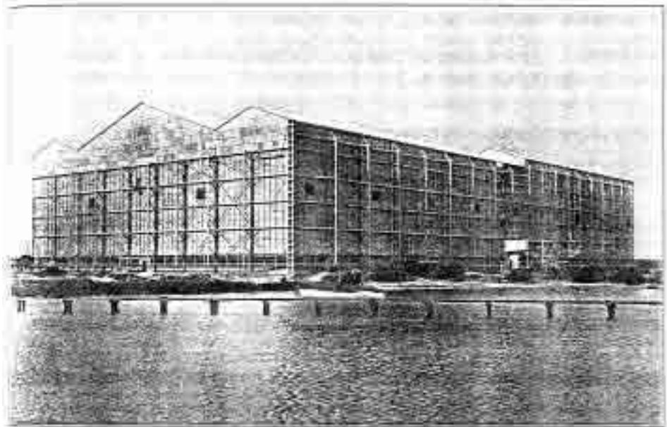
FIGURE 2.—Exterior view of the tunnel.
