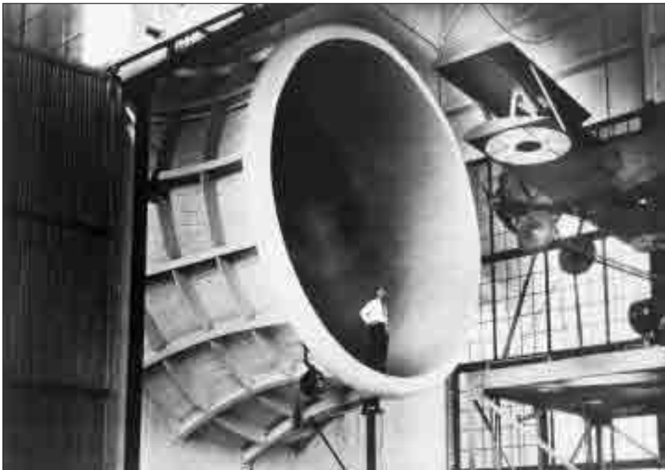
NACA Langley's chief of aerodynamics, Elton W. Miller, inspects his researcher's installation of a Sperry M-1 Messenger airplane into the lab's new Propeller Research Tunnel (PRT) in early January 1927. This was the first complete, full-scale airplane ever to be tested in a wind tunnel in the United States. NASA Image #L-01892 (LaRC)
