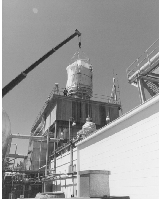
Figure 14. MHTB installation in test stand 300 vacuum chamber—beginning.
