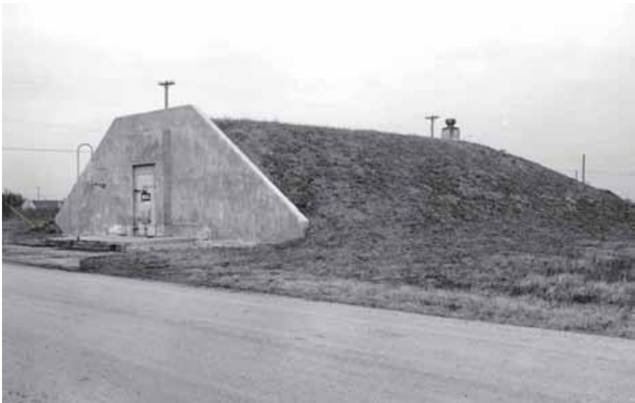
Image 13: One of ninety-nine bunkers used to store powder at Plum Brook's southwest corner. These structures function today as naturally climate-controlled warehouses for federal records. Courtesy of Corps of Engineers, U.S. Army. (No. 21762, 1944)
