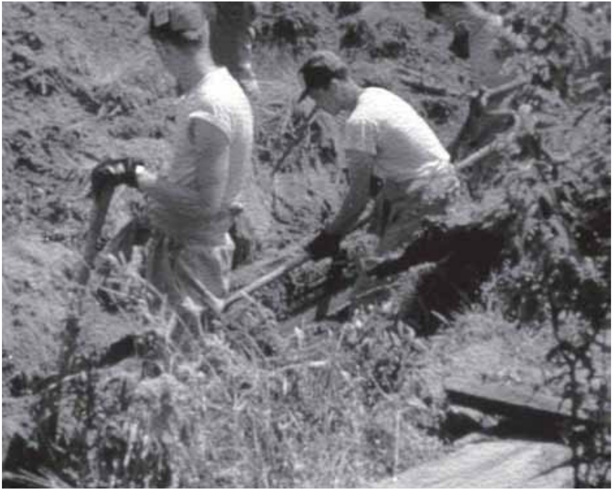
Image 20: Workers dig up transit lines, flumes, and buried TNT at Plum Brook. The explosive remains were then detonated safely elsewhere. Despite claims that there would be no long-term damage to the land, by 1948 it became evident that the Plum Brook site had suffered considerable contamination. During the early 1950s the land became a subsidiary of the nearby Ravenna Arsenal and was subjected to even more contamination. The NACA attempted to clean up the area in the mid-fifties. The United States Army Corps of Engineers is still working on the project today. (1956) (NASA C-2003-826)
