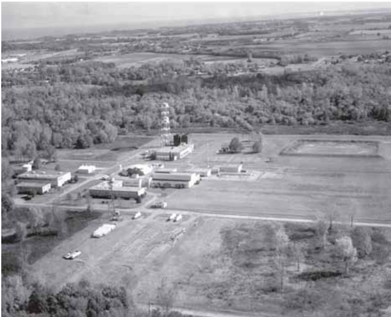
Image 126: For almost thirty years, the facility remained sealed and constantly monitored to ensure that no contamination escaped. However, aesthetic maintenance was not as important, as shown by the peeling paint on the once shiny reactor dome. (1981) (NASA C-1981-4957)
