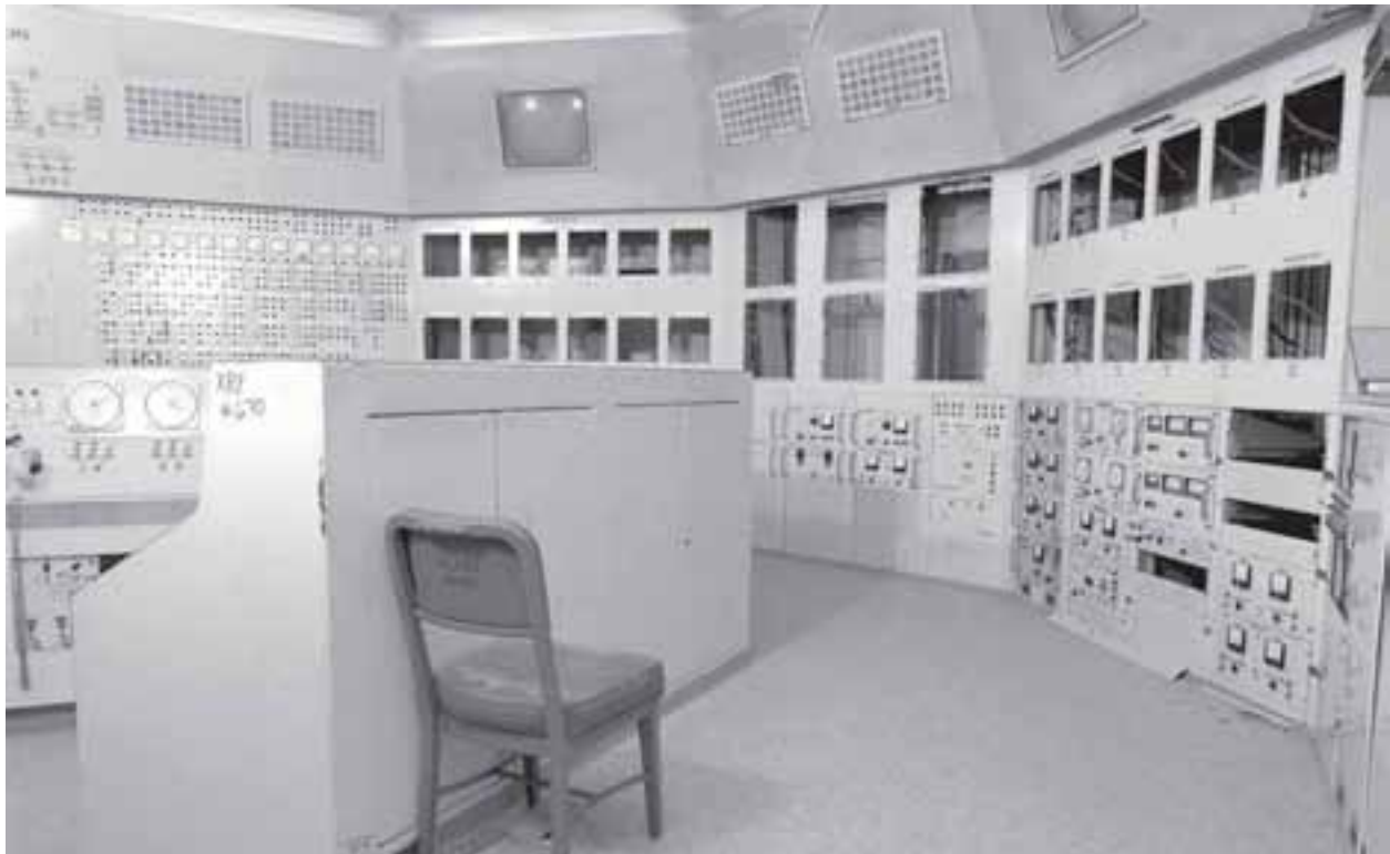
Image 131: The Plum Brook reactor control room in 2001, stripped of a significant amount of its instrumentation. (NASA C-2001-01221)
