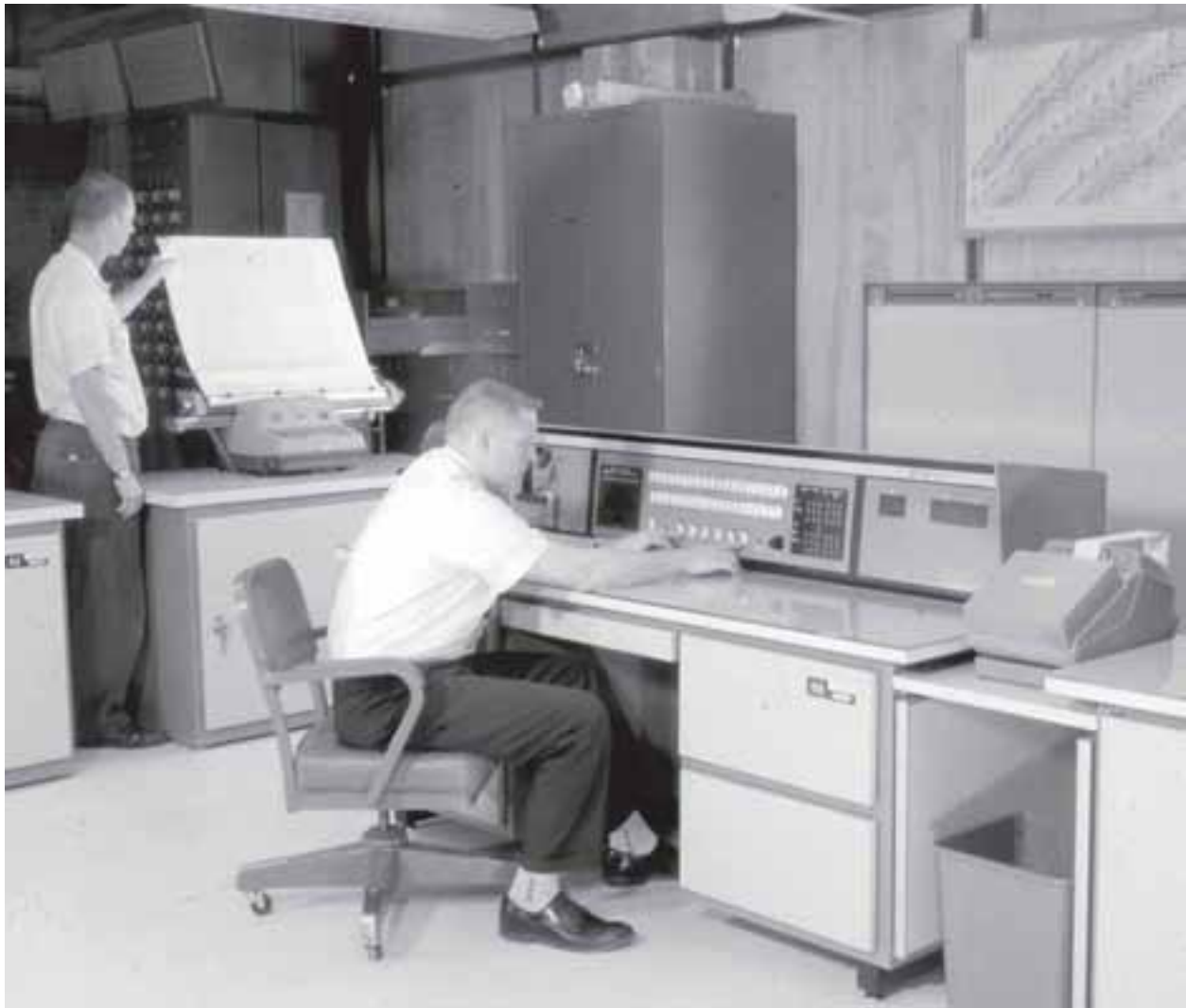
Image 93: The experiment control room, located directly below the reactor control room, contained various monitoring equipment. In this photo, Johnny Miller examines the Experiment Data Logging and Alarm System, which recorded all events during the operating cycles of the Plum Brook reactor in minute detail. Earl Boitel, seated, checks data input sources. (1964) (NASA P64-0713)
