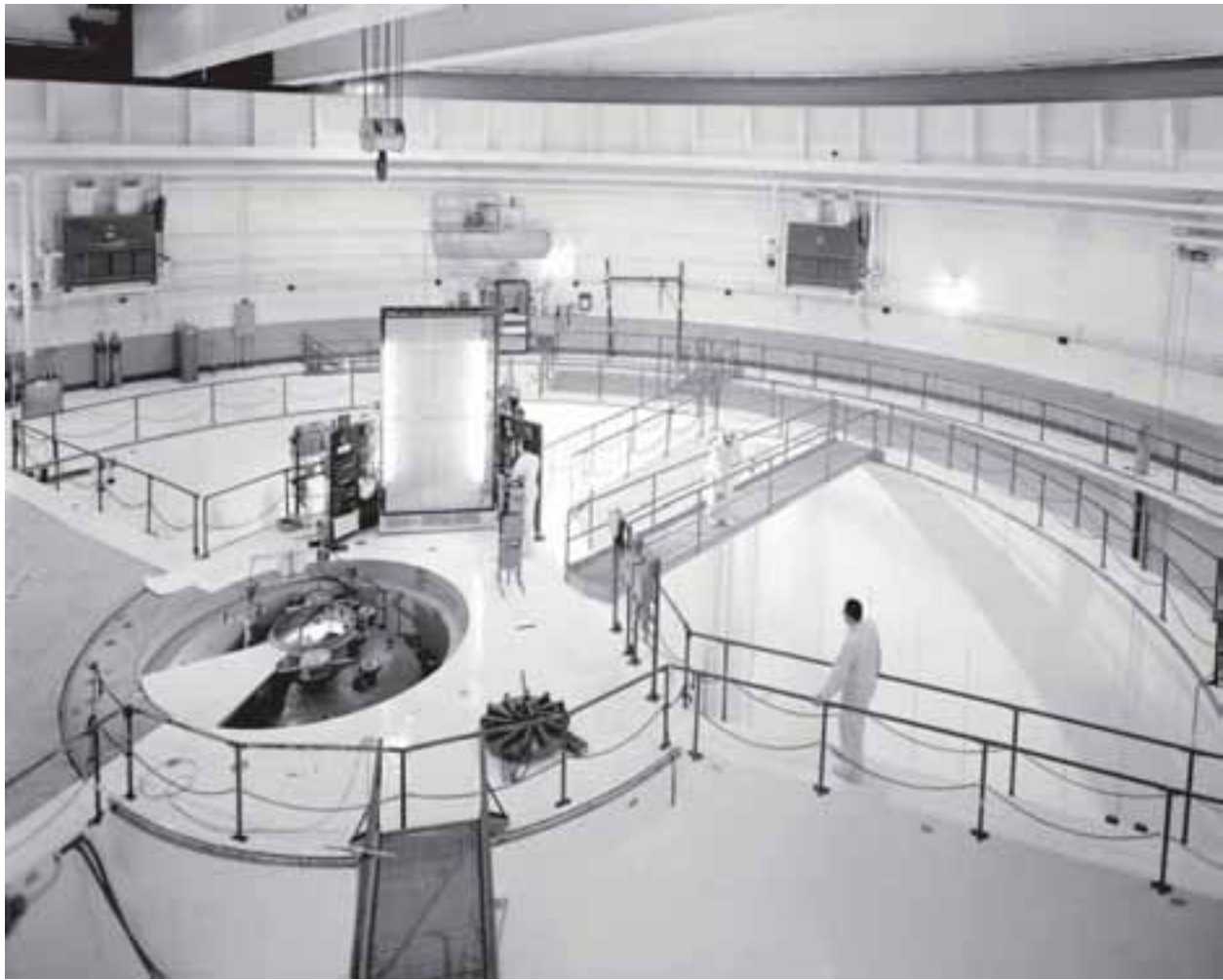
Image 63: The lily pad area atop the reactor pressure tank. For over ten years, engineers subjected materials to radiation within this vast, cathedral-like containment vessel. In this picture, the shrapnel shields have been removed from over the pressure tank and the hatch has been removed and placed on the lily pad, revealing the open reactor tank. Monitoring was performed and experimental equipment was often assembled in this area. (1961) (NASA C-1961-55851)
