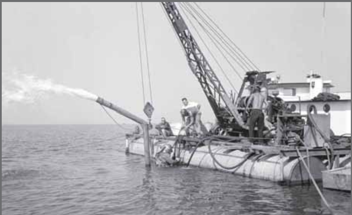
Image 52: A diver emerges after working on the Plum Brook water pumps in Lake Erie. Divers had to flush the intake line and clear it of mud, silt, and debris regularly. (NASA C-1961-58167)
