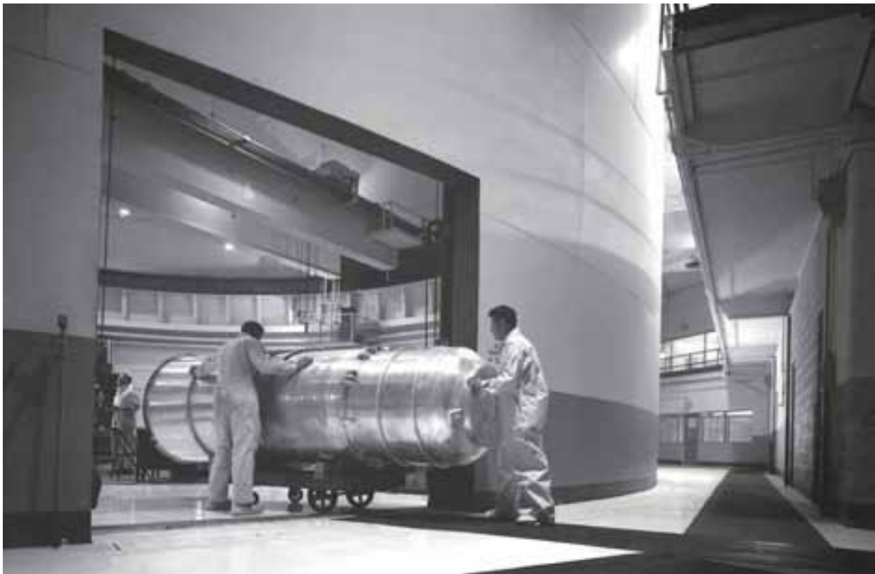
Image 103: Technicians wheel a large “thimble” containing experiments for irradiation into the containment vessel through the truck door. When the reactor was shut down and the protection of the containment barrier could be broken, this door was the only way large items of equipment and hardware could be taken in or out of the containment vessel, utilizing fork lifts if necessary. (1961) (NASA C-1961-55811)
