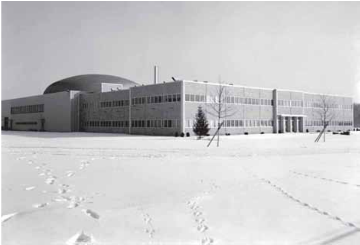
Image 125: After its mothballing in 1973, the reactor went silent. It was visited only by the numerous deer in the area and a skeleton crew that continued to monitor the facility during the standby period. (NASA C-1961-55643)
