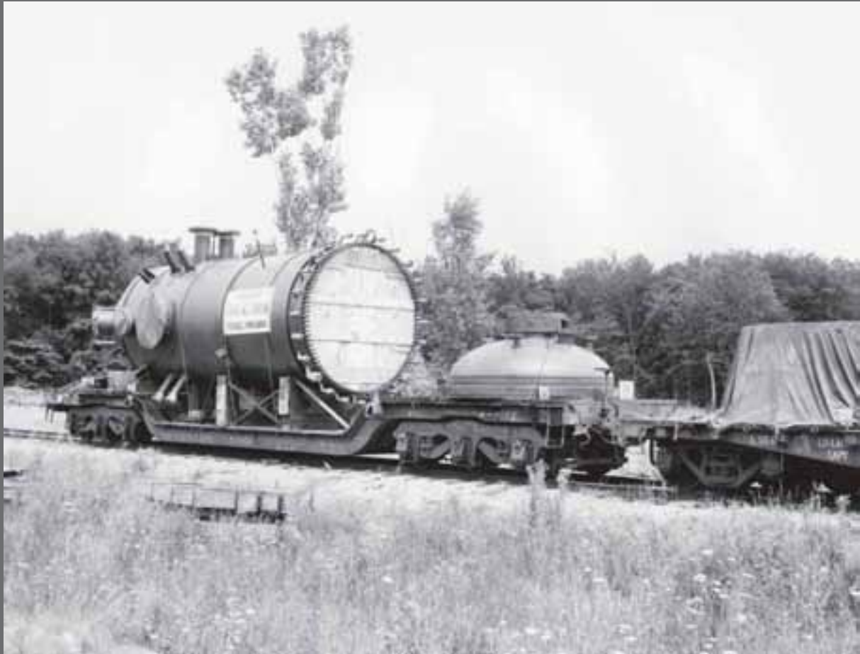
Image 45: The pressure tank was shipped to Plum Brook via railway, and transported to the reactor facility on a flatbed truck. The tank was then rolled to a crane, which lifted it into place at the center of the unfinished quadrant area. Several pipes jutted out from the tank. These “test holes” would be used to transport experiments to the reactor core for radiation during its operating cycles. (c. 1959) (NASA C-2003-833)
