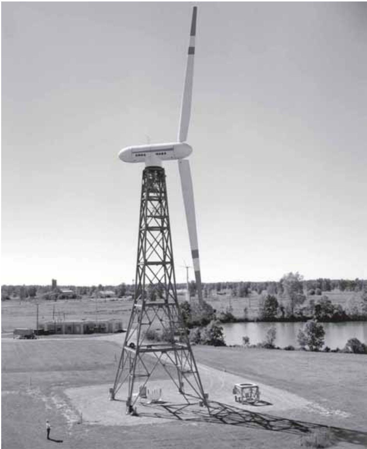
Image 124: Spurred by the energy crisis, NASA, and the Energy Research and Development Administration (ERDA) installed this large 100-kilowatt wind turbine for alternative energy research at Plum Brook. The 100-foot tower supported two sixty-two-foot blades, which could reach forty rpm in eighteen-mph winds. When the Plum Brook reactor shutdown was announced, Congressman Mosher and others endeavored to find alternative uses for Plum Brook Station. The wind turbine was one of the few successful programs on the station in the 1970s and 1980s. By the late 1980s, several of the testing sites at Plum Brook were reactivated and remain in operation today. (28 September 1976) (NASA C-1976-3906)
