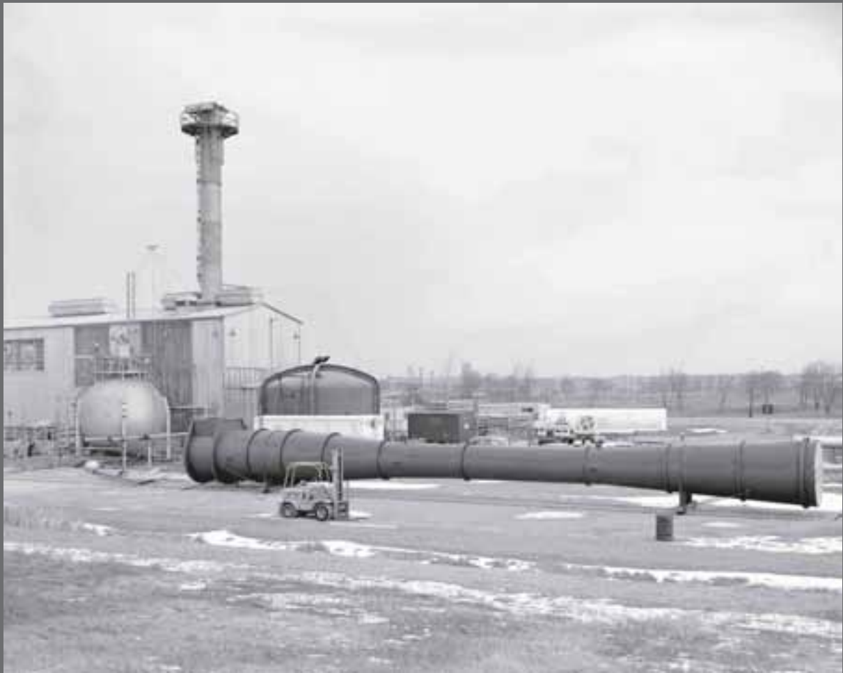
Image 108: The Hypersonic Tunnel Facility was capable of creating air velocities and temperatures that simulated flight speeds of seven times the speed of sound, at an altitude of 120,000 feet. (1969) (NASA C-1969-00725)
