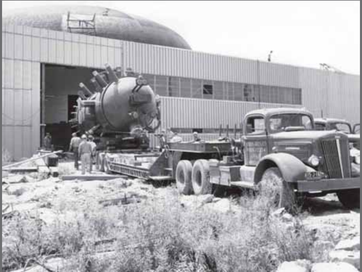
Image 46: The pressure tank delivered by truck. (NASA C-2003-834)
