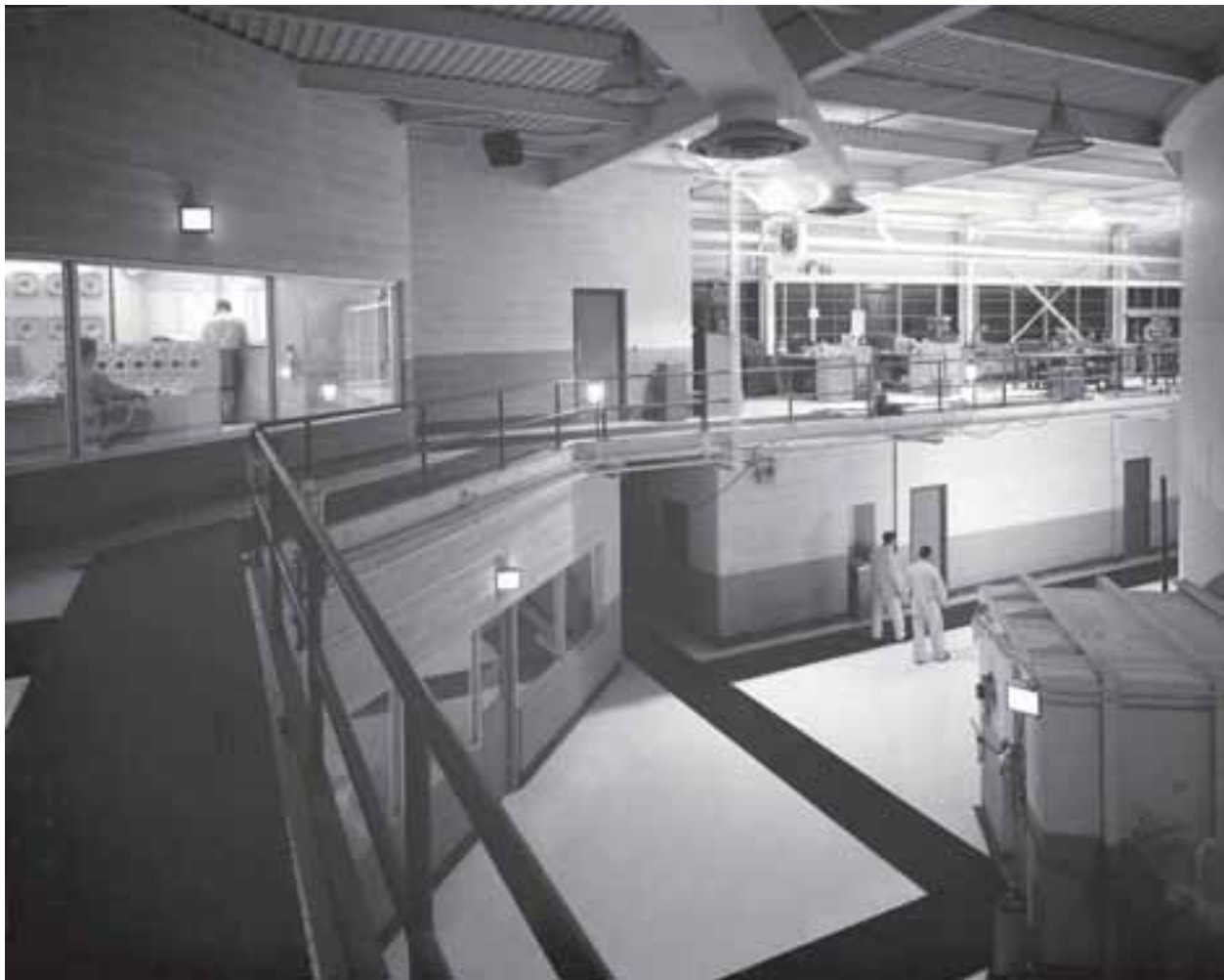
Image 65: The area just outside the containment vessel airlock (bottom right). The reactor control room on the second floor is visible to the left. The experiment control room is directly below it on the first level. On the second level to the right is a workarea that was later segmented and enclosed for office space. In this picture, three of the “Reactor On” signs are illuminated, indicating that the reactor is in operation. (1961) (NASA C-1961-55812)
