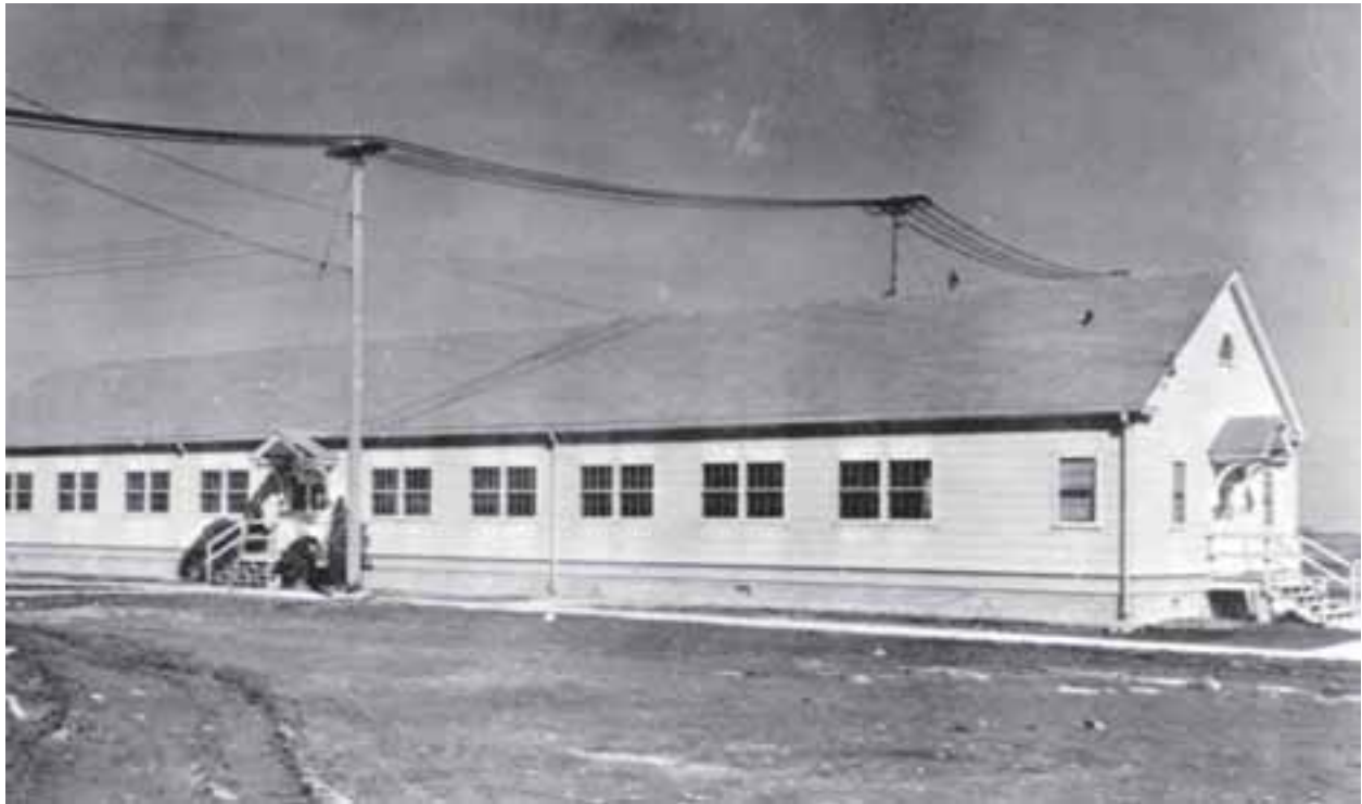
Image 11: The Plum Brook cafeteria building, a typical Ordnance Works structure. Plum Brook's ordnance buildings were built for functionality, not style. Although these structures were built to last five years, many survived much longer, and this building is today used by the Perkins School District. Courtesy of Corps of Engineers, U.S. Army. (No. 3-42, 1944)
