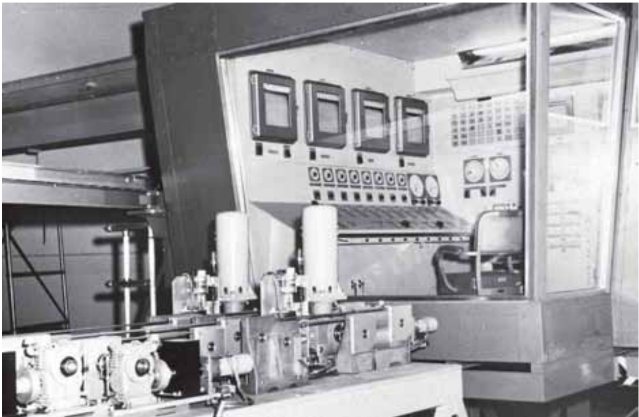
Image 71: The control room for the Mock-Up Reactor was perched directly above its core. The large windows allowed the operators to view the controls and monitors, as well as the activity in the core below. (NASA PS63-0008)
