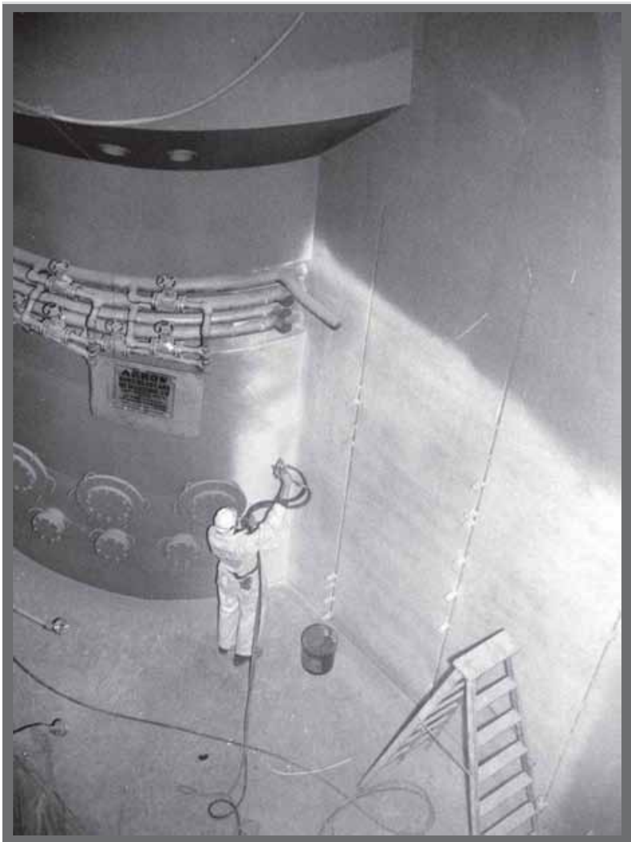
Image 50: A worker spray paints one of the quadrant walls and a shielding wall surrounding the reactor pressure tank. The quadrants were twenty-five to twenty-seven feet deep and filled with water. The water provided shielding for the radioactive materials that were transported along the canal basin. (NASA C-2003-837)
