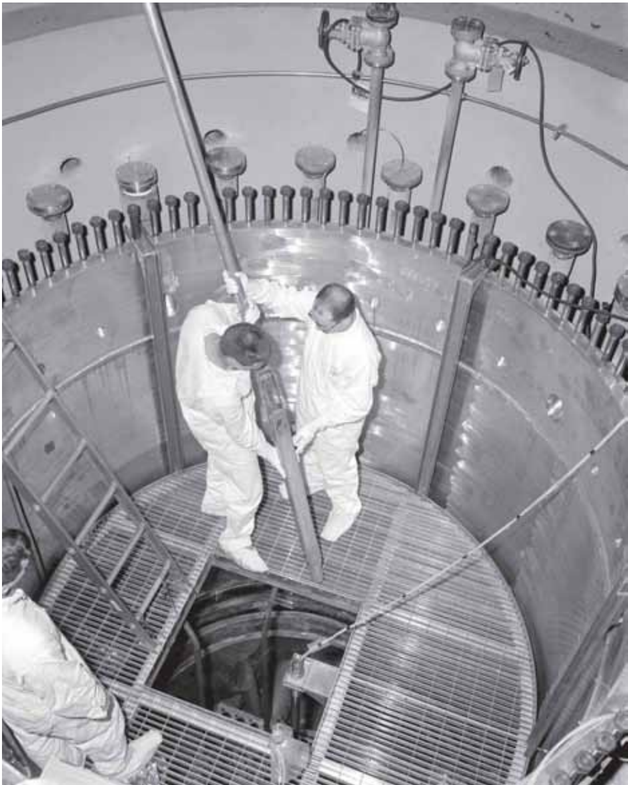
Image 61: Jack Crooks (right) and Jerold Hatton work inside the reactor tank in preparation for the initial startup of the Plum Brook Reactor. They are inserting dummy fuel elements into the core as part of the final hydraulic testing. (1961) (NASA C-1961-56897)
