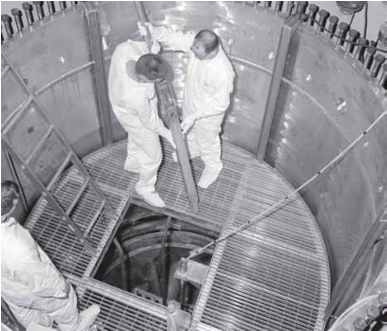
Image 68: Three technicians work on the core, inside the pressure tank, during one of the shutdown periods. Experiment cycles varied greatly. Some lasted months, while others only days. Each cycle consisted of two parts—the shutdown portion and the power portion. The shutdown periods were used to change fuel, perform maintenance, and work on experiments. (NASA C-1961-56897)
