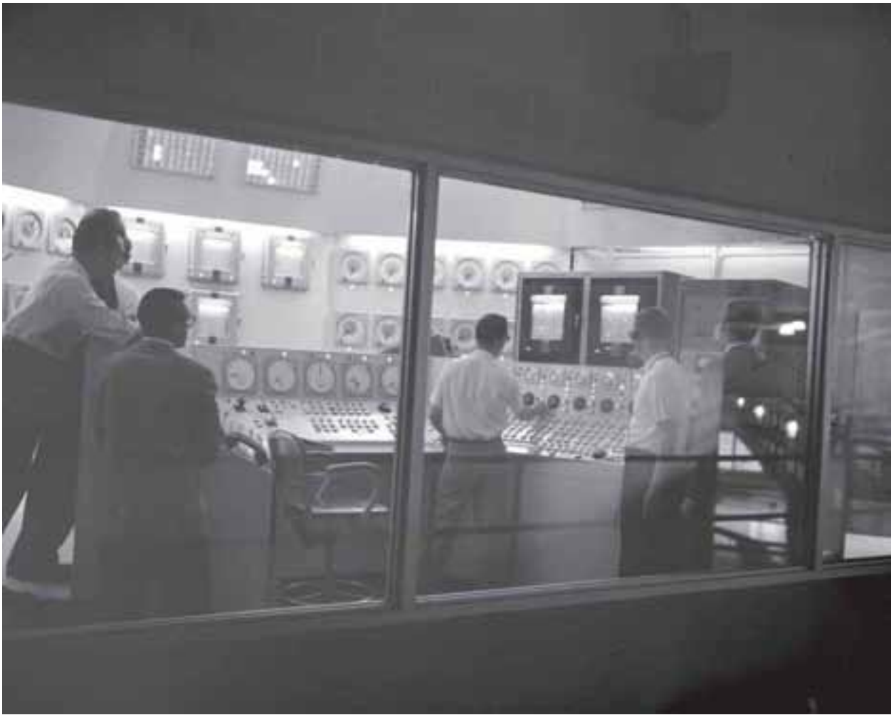
Image 62: Harold Geisler takes the Plum Brook reactor critical for the first time on the evening of 14 June 1961. This first self-sustaining chain reaction was conducted at very low power. It wasn't until the following April that the reactor reached its full potential of sixty megawatts. By July 1963, the reactor had completed its first experimental cycle while critical. (NASA C-1961-56899)
