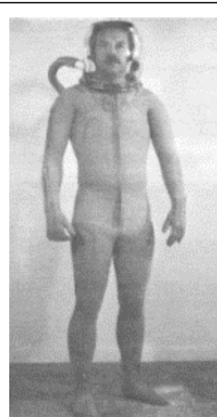
Figure E-1. The Annis-Webb mechanical counter pressure suit concept from the 1960s.
