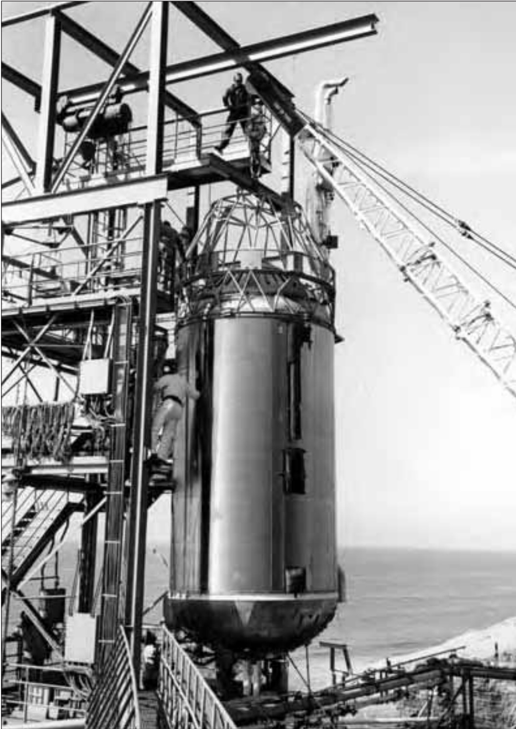
Centaur is raised into the "J" Tower for testing at Point Loma, early 1960s. (Courtesy of Lockheed Martin)
