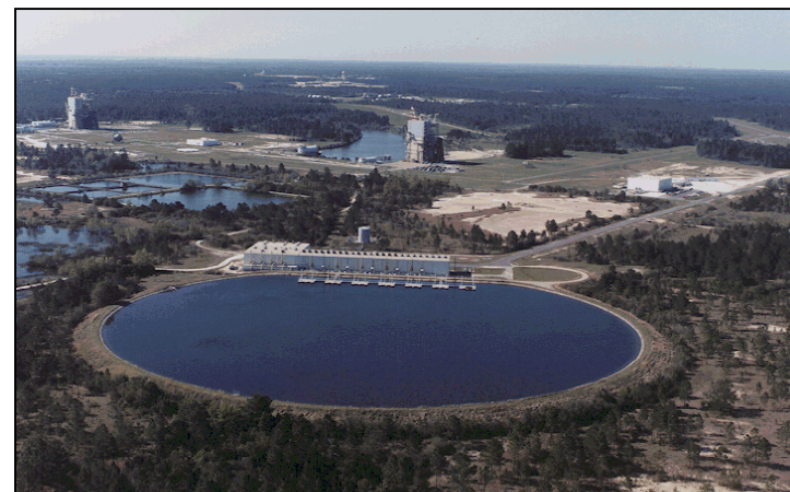
High Pressure Industrial Water (HPIW) 330,000 gpm
