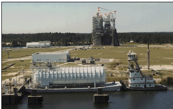
Cryogenic Propellant Storage Facility Six (6) 100,000 Gallons LOX Barges Three (3) 240,000 Gallons LH Barges
