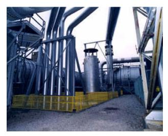
The Reduced Noise Gas Flow Design Guide enables the development and implementation of noise-control strategies such as this silencer, which reduces the noise generated by the multiple pressure relief valves associated with Glenn's Central Process Air System. This system provides high-pressure processed air and exhaust to support Glenn's experimental facilities.
