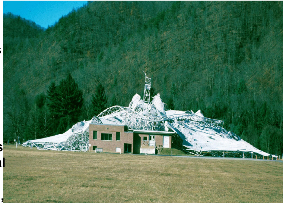
NRAO's 30-year old 90m Antenna in its Ultimately Relaxed State: Higher duty cycle → Metal fatigue
