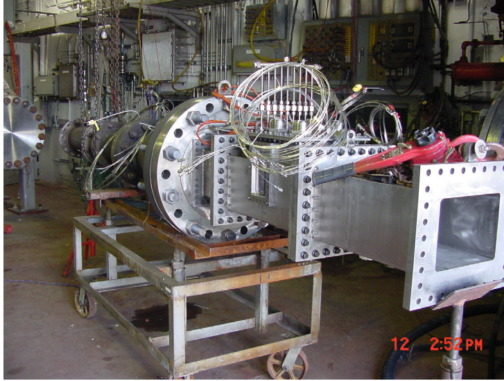
Figure 4.—Combustion Rig Being Installed into the GE Facility.
