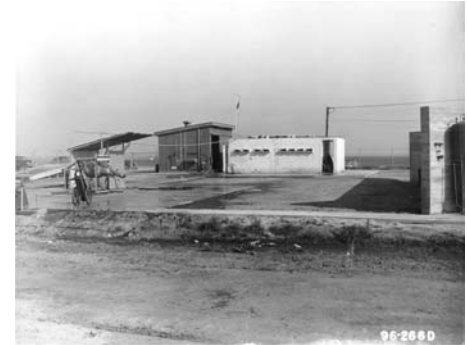
NAA LAX Parking Lot Control Center - 1947
