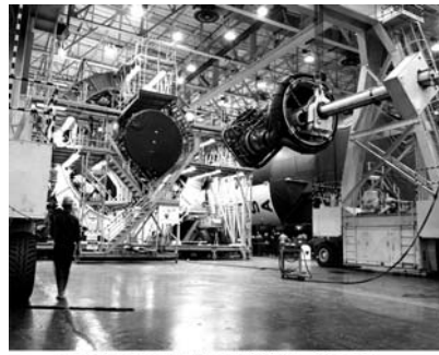
F-1 Engine Horizontal Installation into S-1C Stage - 1965 (4 of 4)
