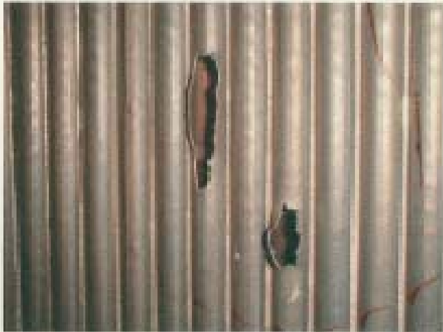
Damage to Regeneratively Cooled Tubes
