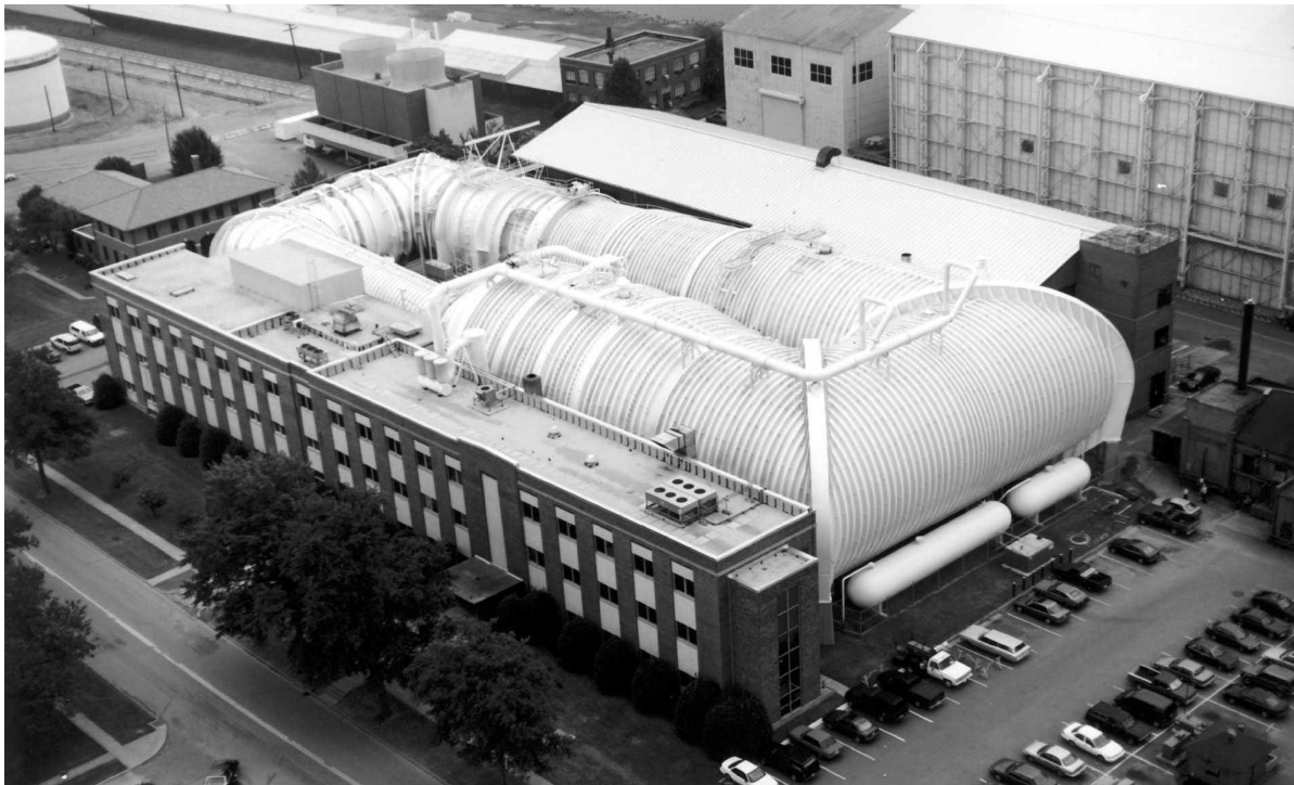
Figure 1. Langley Transonic Dynamics Tunnel (TDT).
