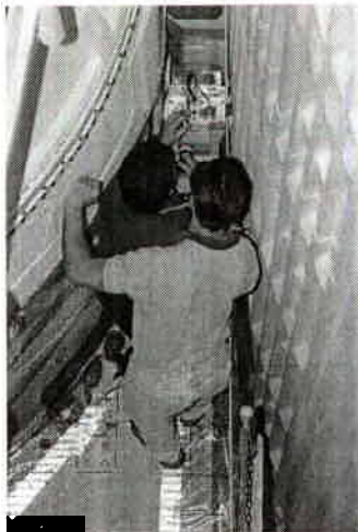
Range Safety Cable Between SRB & ET
