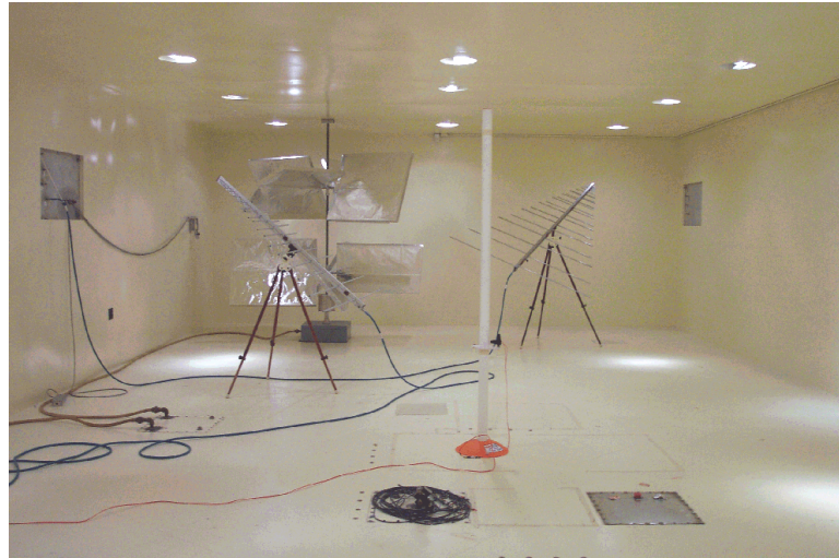
Figure 3.2-1: Inside reverberation Chamber A.
