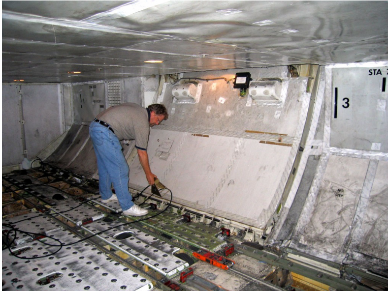
Figure 4.1-6: Scanning the transmit antenna along cargo door seam of a B747-422 aircraft.
