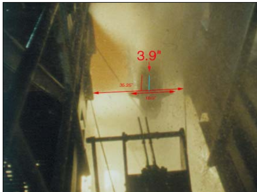
Figure 2.2 GH2 Vent Arm South of Center Contact with the Deceleration Cable During Latchback (Camera E39)
