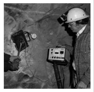
Deep within a mine shaft, Dr. Joseph Heyman looks on at early testing of NASA's bolt elongation monitor. Heyman is monitoring mine roof bolt preload during a test to compare the P2L2 data to that of a pressure plate. The tests demonstrated that, with the P2L2, each bolt could become its own precision load monitor.
