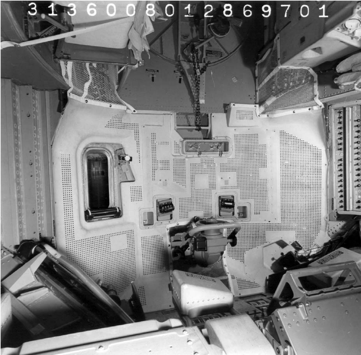
Photo 25. View of Overhead LM Ceiling
