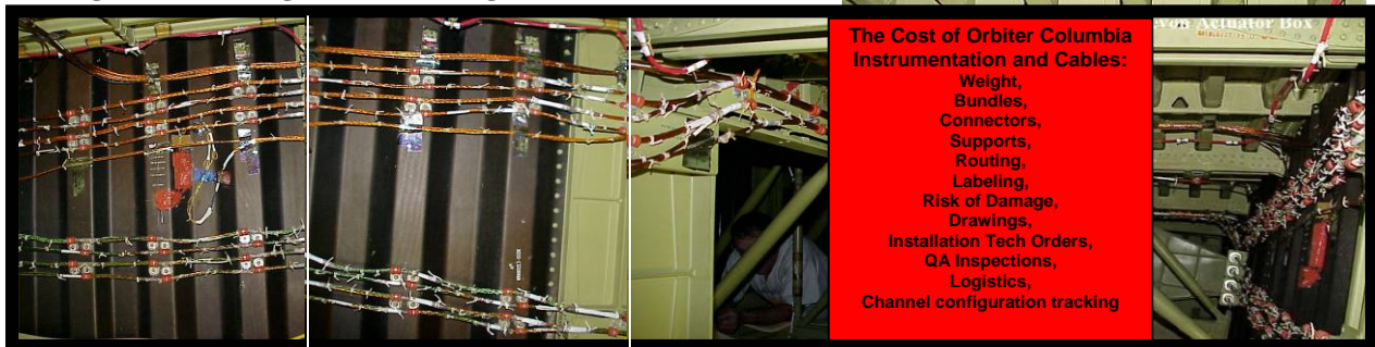
Figure 1: Wiring Inside the Wing of the Orbiter Columbia costs more than length and weight.
