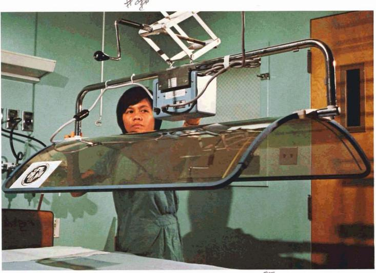
The heated transparency is also a feature of a new Sierracin-Cavitron product, introduced last year, the Stanford Transport Incubator System. Developed by a team of medical and engineering personnel at Stanford University Medical Center, this unit meets a need for transporting seriously ill infants by airplane or ambulance to a specialized care facility.
