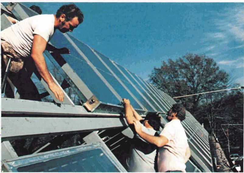
beneath the building. In operation, water is directed through the solar collectors, heated by the sun and routed back to the storage tank, from which it is pumped into the building's regular hot water heating system as needed. During periods when the sun is obscured by clouds, the existing oil furnace automatically takes over the heating job.
