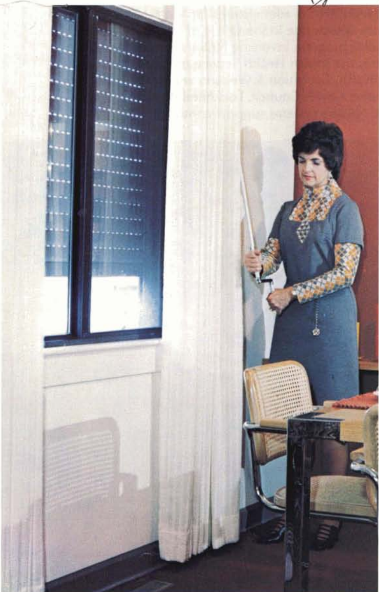
The window at left has thermal shutters, which are rolled up or down by a crank handle. When closed the Venetian blind-type shutters form an exterior window seal to keep heat in or out as desired.
