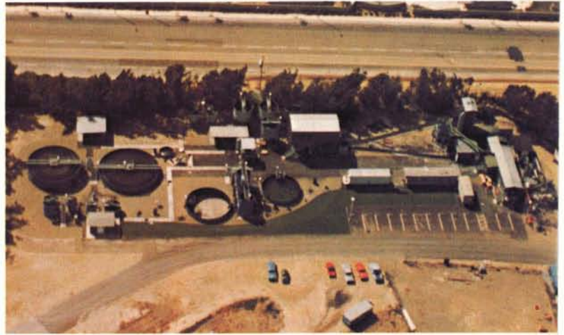
This 1,000,000 gallon per day pilot plant in Orange County, California is evaluating a NASA-developed pollution control technique known as ACTS (Activated Carbon Wastewater Treatment System). ACTS is based on the knowledge that activated carbon is an effective agent for treating sewage, and solid sewage, in turn is an excellent material from which to make carbon. In the plant, filtered solid sewage is burned (without oxygen) to produce activated carbon and the carbon is used to treat the wastewater. The process yields water as clean as that resulting from conventional methods, but at significantly reduced cost.
