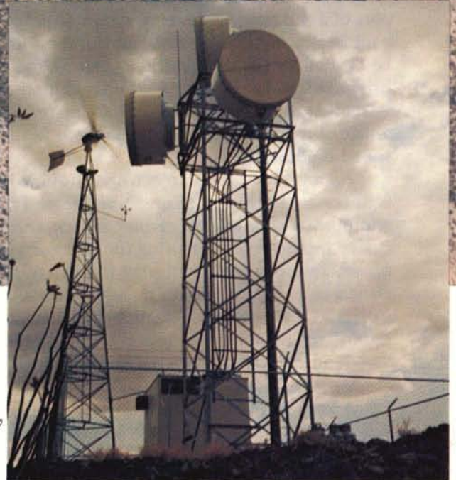
A major element of STARPAHC's space-derived telecommunications network is this microwave station on Quijotoa Mountain, near the center of the Papago reservation. The station relays TV, voice and medical data between the Sells hospital, the Mobile Health Unit and a fixed clinic in the town of Santa Rosa.
