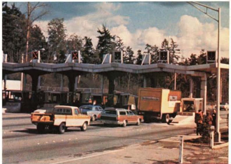
*These toll booths, at the Evergreen Point Bridge near Seattle, Washington, have air purifiers whose design profited from NASA "clean room" airflow technology. The booth's airflow system retards infiltration of contaminated air and decreases the toll collector's inhalation of engine exhaust fumes.*
