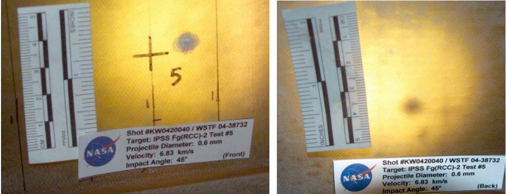
Figure 61: Fg(RCC)-2 Shot #5 Backlit Impact Damage (Left: Front Side, Right: Back Side)
