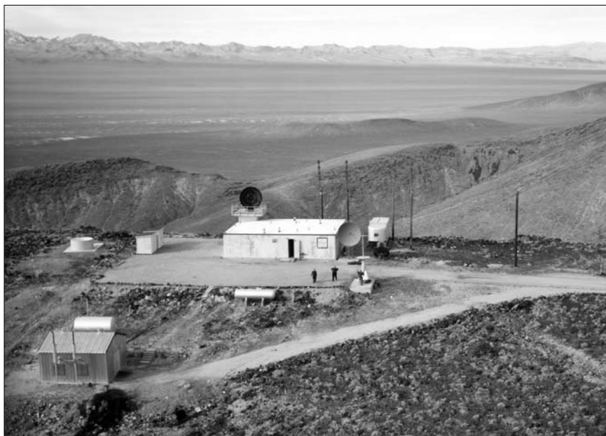
The High Range stations were positioned on top of mountains to provide the best look angles for the radar and telemetry receivers. The Beatty, Nevada station was closed when the X-15 program ended and nothing remains at the site except for the concrete slabs where the buildings once stood. (NASA)
