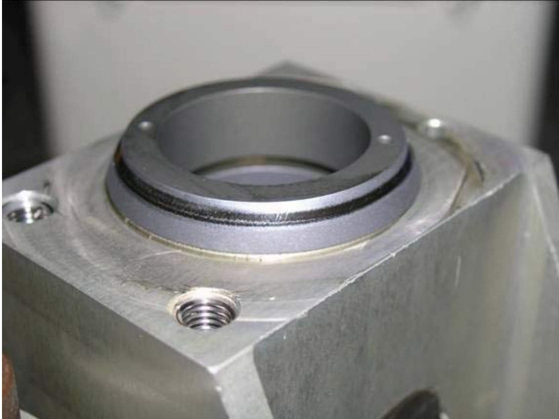
Figure 7. S/N 006 male shear tie, showing acceptable wear pattern
