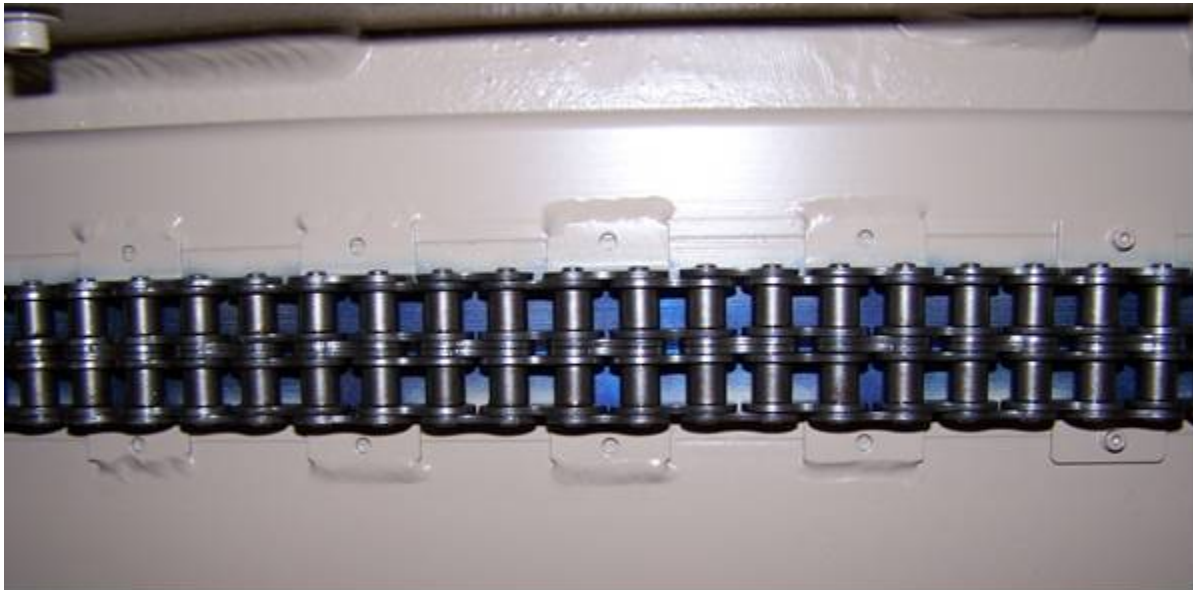
Figure 314. The Drive Chain Was Installed On The Rotating Ring, With The Majority Of Pads Being Welded.
