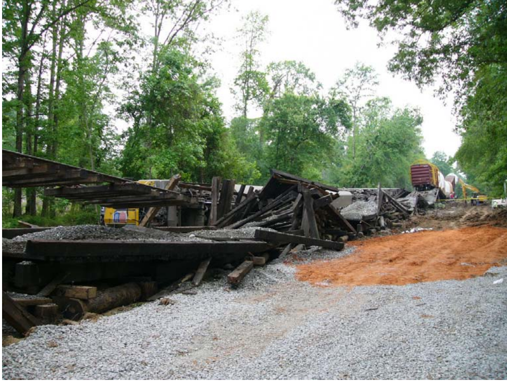
Figure 4. Collapsed Trestle
