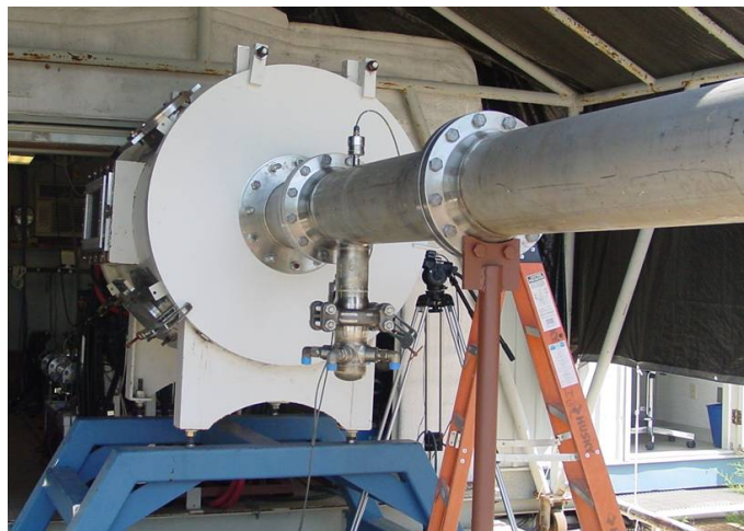
Figure 16. Installed test section and ejector pump.
