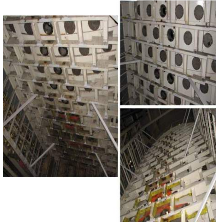
External chamber modifications – removal of solar simulator structures
