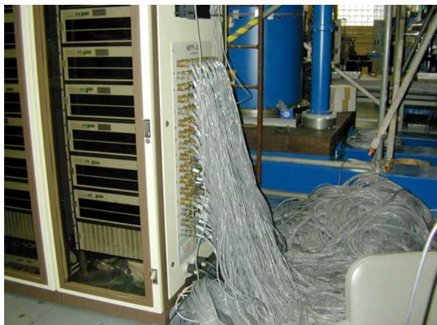
Figure 1. Photograph of the cabling required to connect 466 foil strain gauges to a wing box test article.
