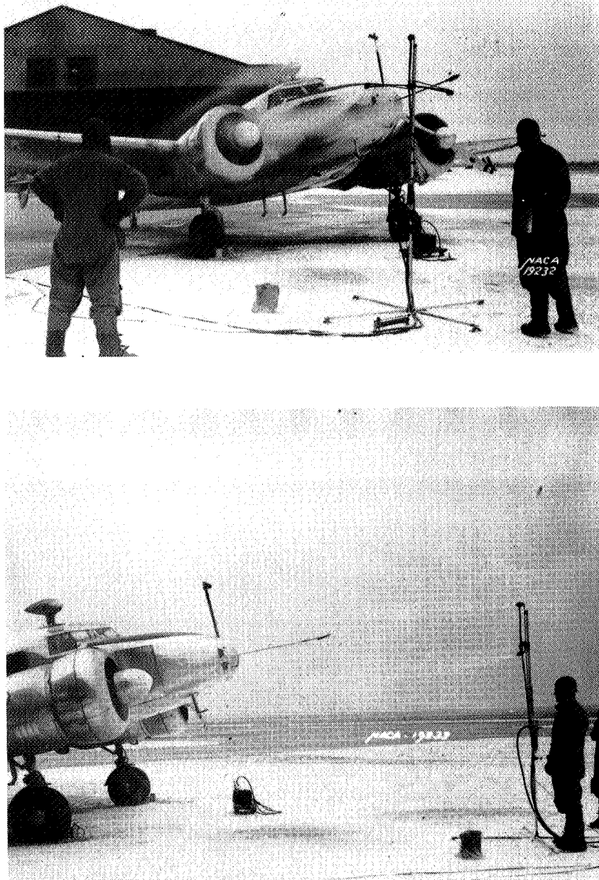
Figure 1.- Two views of Lockheed 12A airplane. Ice was formed on the rotating propellers of the airplane while on the ground.
