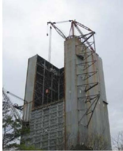
**Figure 10.** The side door was opened on Test Stand 4550 and the roof panels were removed for the first time in 29 years this past April.
