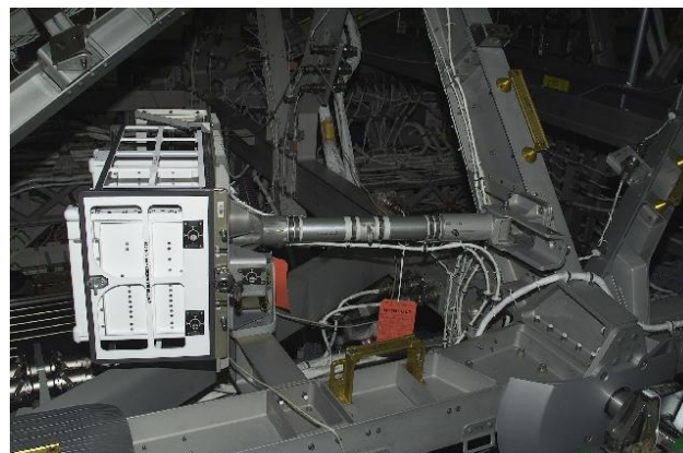
Figure 2. EVCPS attached to the S0 Truss
